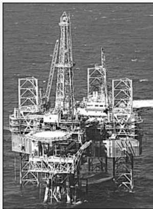
Oil rig in Bombay High.
